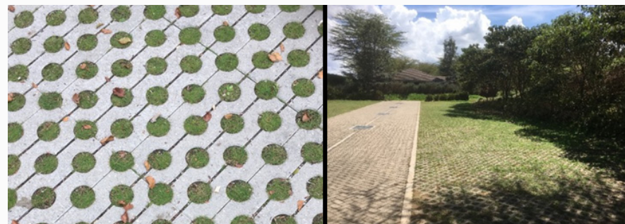
Figure 9 examples of permeable paving, the example on the right is found in Naivasha, Kenya.
