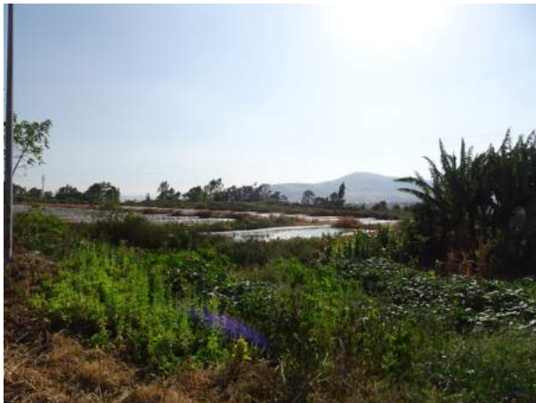
Figure 18 Sludge drying beds at Kality WWTP with testing plots of dried sludge at the righthand side (Source, field visit WWX 1 November 2021)
