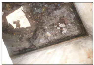
Figure 1-7: Village communal septic tank full of sand and sludge (UNICEF-oPt/2012/Spit)
