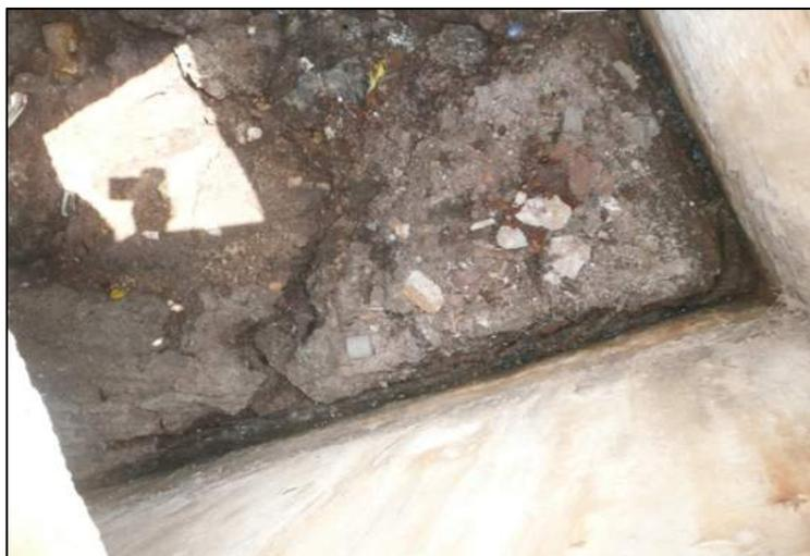
**Figure 1-7: Village communal septic tank full of sand and sludge (UNICEF-oPt/2012/Spit)**
