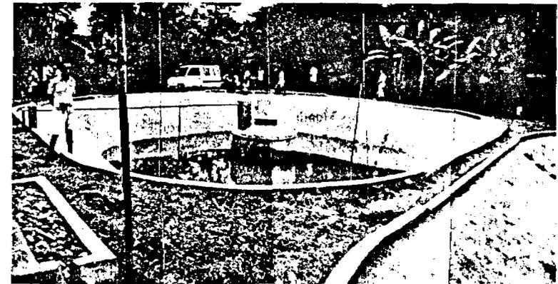
Fig. 2. The slow sand filter. The collection well is seen in the middle and the pole valve is on the right.
