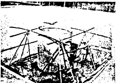
Fig. 8. Setting up of the mould for the collection well.
