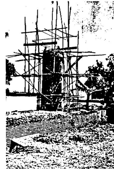
Fig. 4. Brickwork tower encased in ferrocement.
