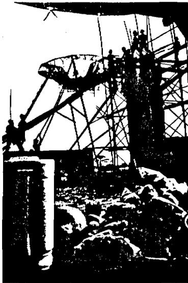
Fig. 6. Tank bottom reinforcement cage lifted manually.
