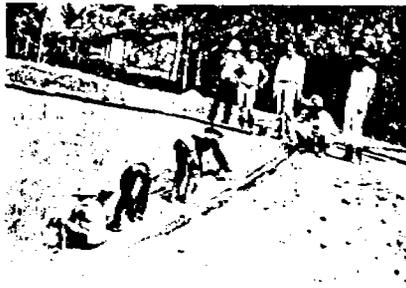
Fig. 6. Plastering the slopes with ferrocement.
