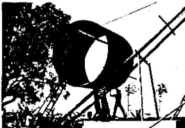
Fig. 7. Formwork of tank rolled up to position.
