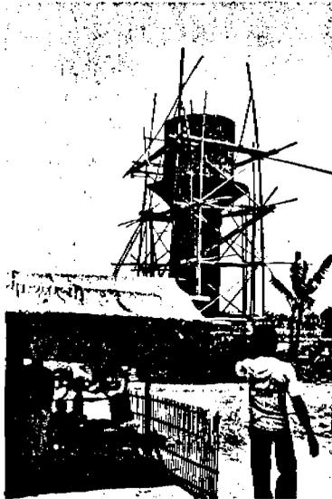
Fig. 8. The water tank after plastering.
