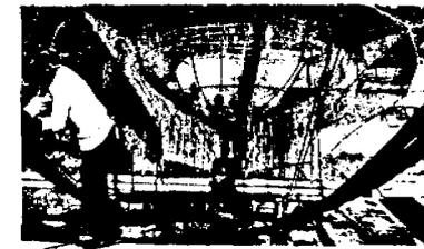
Fig. 5. Saucer shaped bottom of tank.
