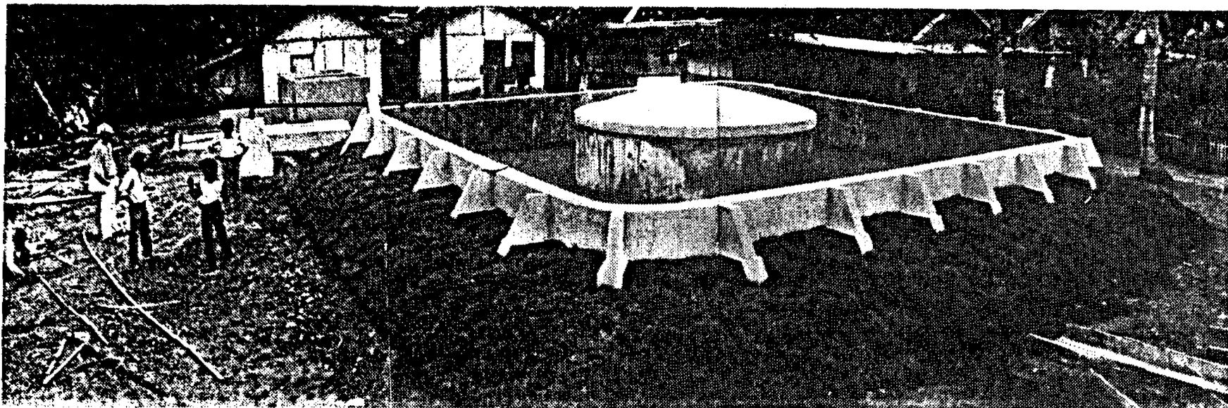
Fig. 8 Slow Sand Filter of Sukareja, a brickwork construction combined with ferro-cement.
